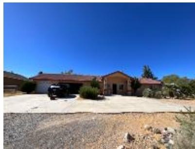
Front view of structure
