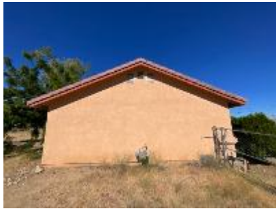
Left side view of structure
