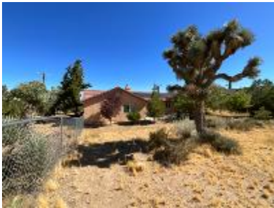
Rear structure view.
