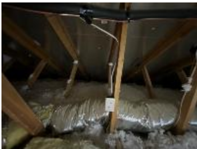
Direct view of air conditioner ducts.
