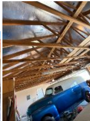
Underside of roof. in garage area
