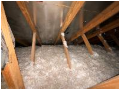
Direct view of blown in insulation
