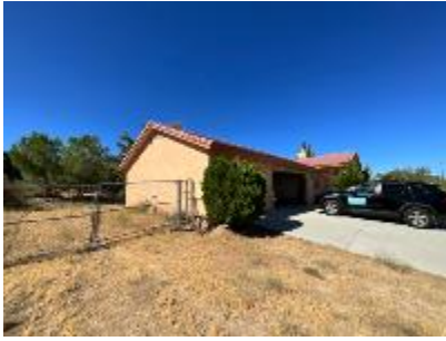
Left side view of structure.
