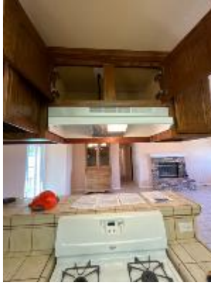
Interior view of kitchen stove Kitchen stove service tag Kitchen ventilation not connected
